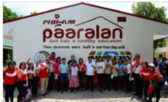
Turnover of one-storey two-classroom building in partnership with ABS-CBN Lingkod Kapamilya Foundation, Inc. in Candau-Ay, Dumaguete City.
